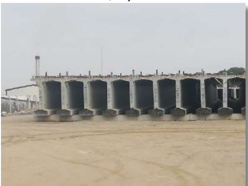
Precast Beams, Kuyucak CCS
